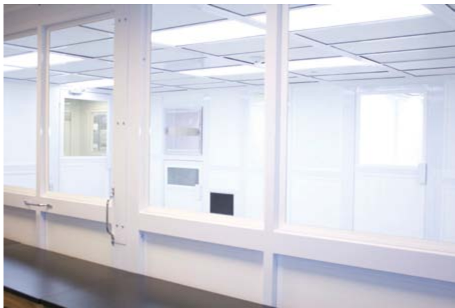
A Grade A/B cleanroom
