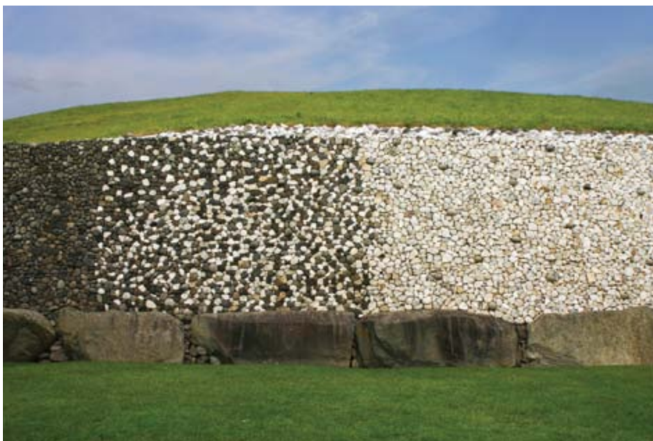
It took at least four generations of people to build the ancient Newgrange tomb in Ireland while today it can be difficult to get someone to follow an SOP twice in two days.
